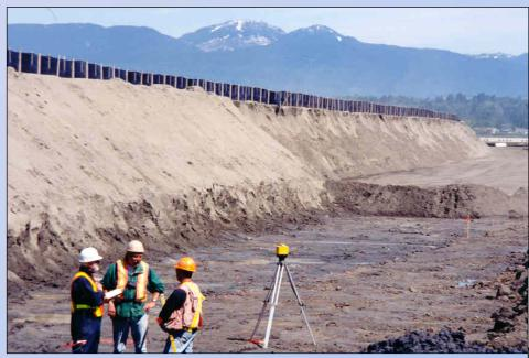
Reuse of Milled HMA on Surface for Protection instead of imported granular
