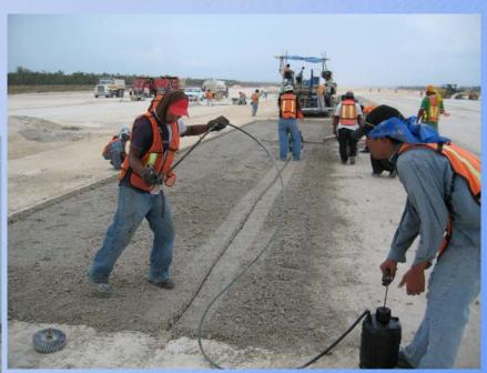
Prevents reflective cracking in HMA surface when cement Contents are high
